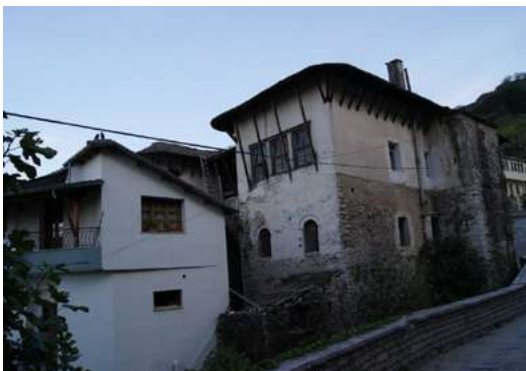
Construction of concrete structures next to monumental houses
