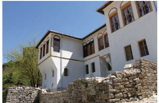
Photos before and after of the Babameto House
